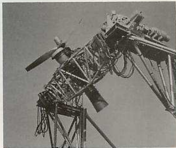
Engines are operated and evaluated on the Variable Attitude Stand.
